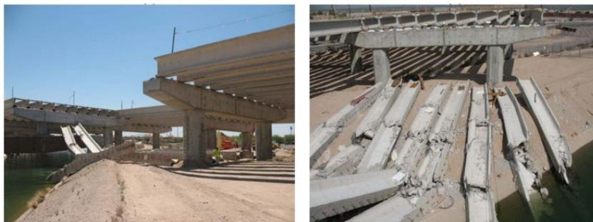
**Figure 1.** Beam collapse in Arizona (EUA). Source: Oesterle et al. [4]
