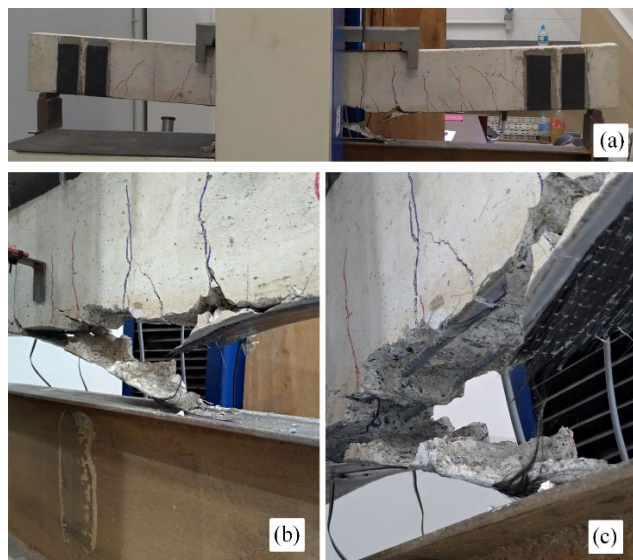
Figure 18. Failure of beam CR63-NI (a); Detail of the rupture and debonding of the CFRP sheet (b); Detail of the non-rupture of the positive reinforcement (c).
