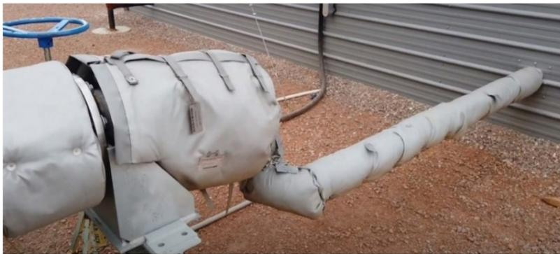
**Figure 8.** Pipe containing the CO<sub>2</sub> that will be injected into the carbonation chamber. Source: [[38]].
