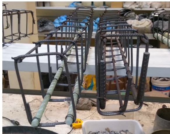
Figure 4. Reinforcement of beams VV37 and VA37.
