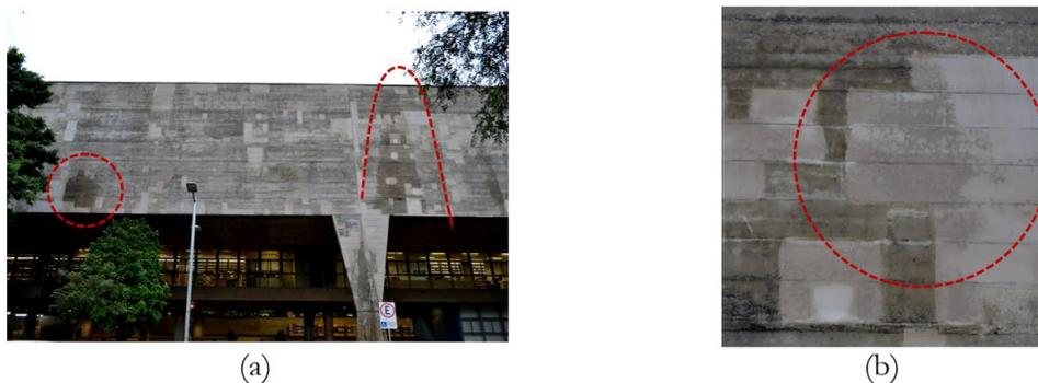
**Figure 4.** Partial views of SW façade: (a) typical moisture stains and (b) noticeable patch repair cracking after rain water penetration (Photos: Authors’ collection, 2017).
