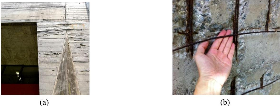
**Figure 2.** Partial view of NE façade: (a) area with concrete disaggregation on pillar P3 and (b) exposure of corroded reinforcement steel (Photos: authors' collection, 2013).
