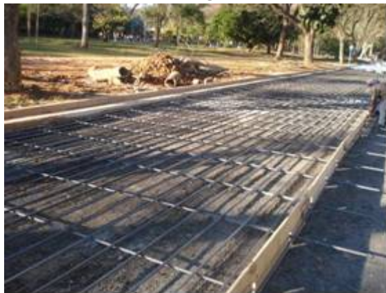
Steel details in Section 1
