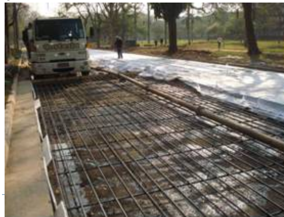
Moist curing (sections 1 and 2)
