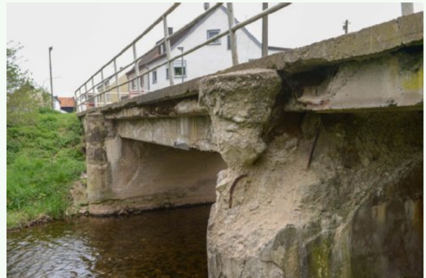
Concrete flaking
