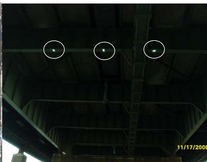
• Reflective Tapes on Bridge Elements
