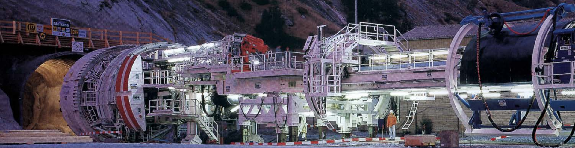
TBM Aberta (Gripper)
