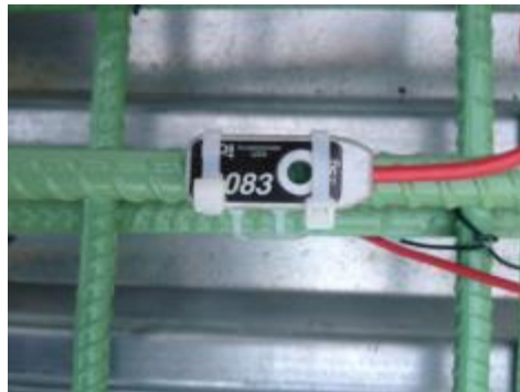
Accelerometers on rebars
