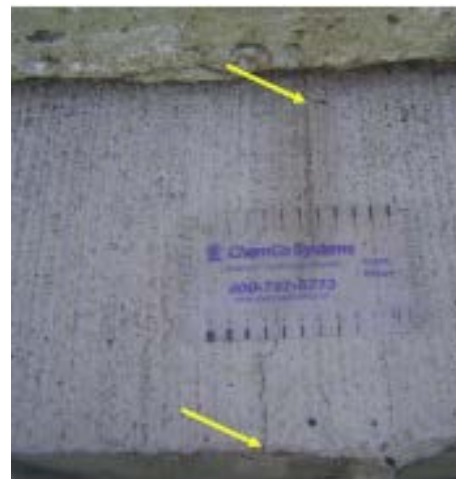
Observed Crack
