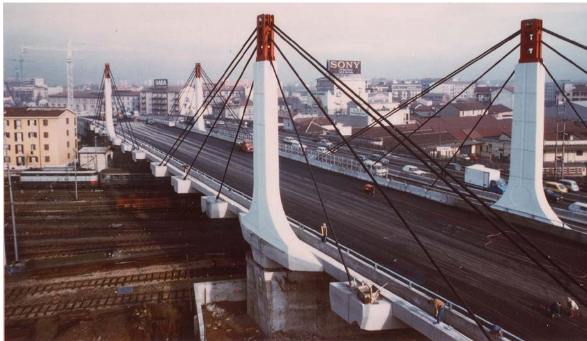
Biondini, F., Frangopol, D.M. & Malerba, P.G. 2006b. Time-variant Performance of the Certosa Cable-stayed Bridge. Structural Engineering International , IABSE, 16 (3), 2006, 235-244
