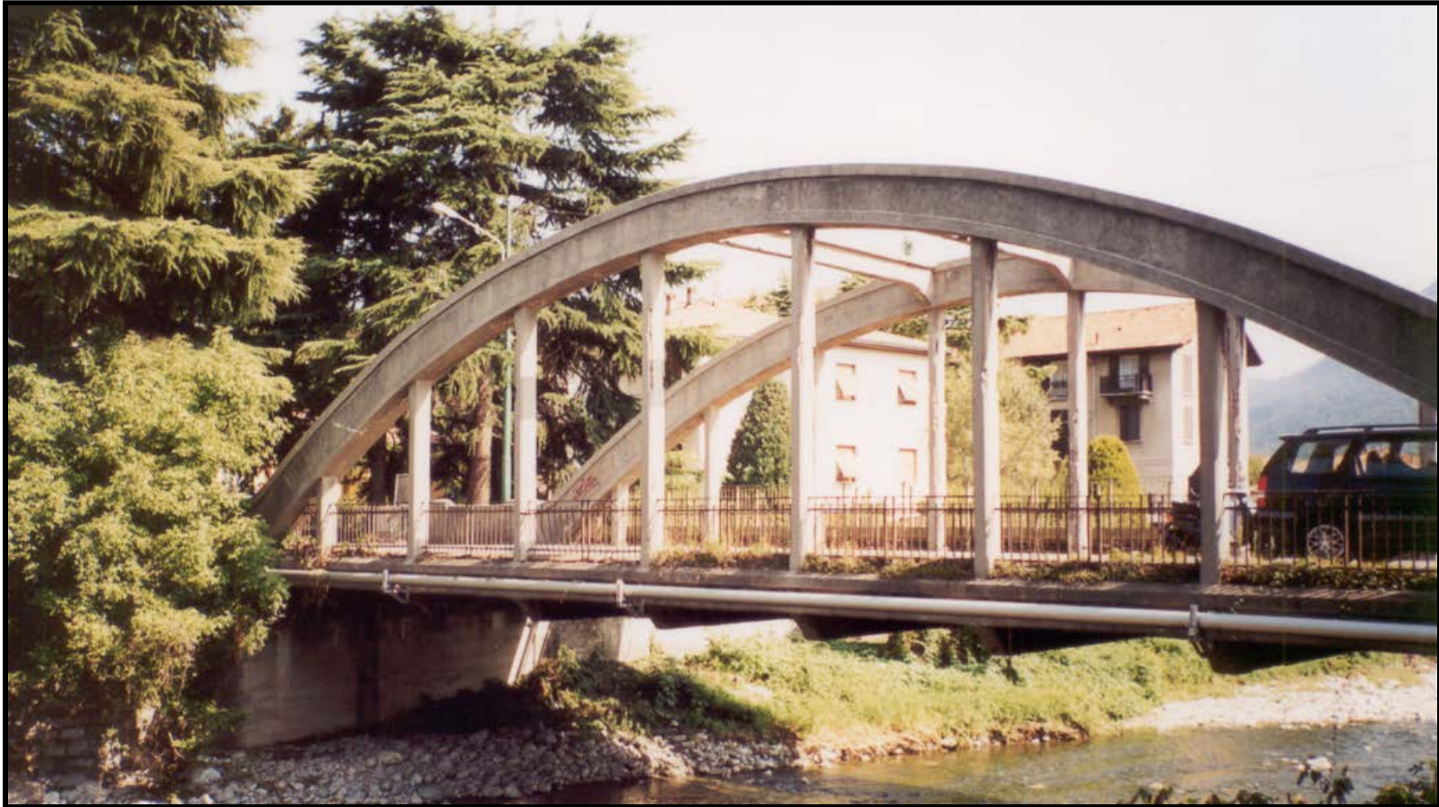
Bridge over the Breggia river (Cernobbio, Italy)
