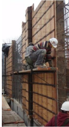
Sheathing & form ties
