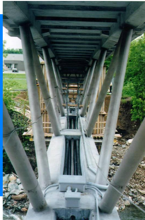
230-MPa RPC foot bridge, Sherbrooke
