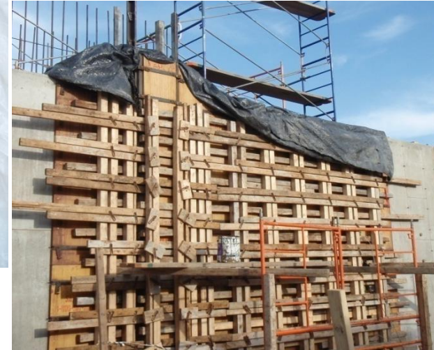
Wall studs & Wales
