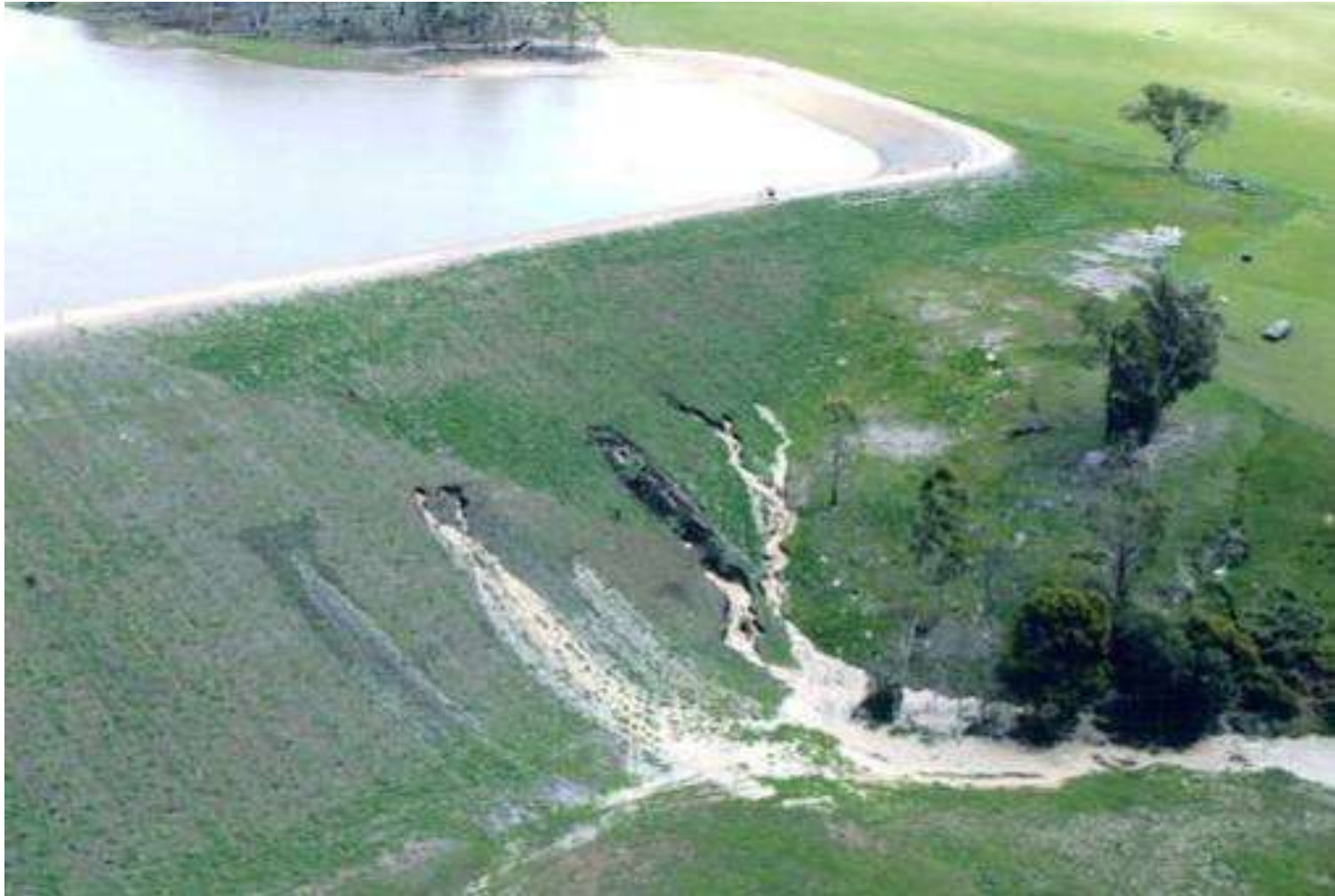
Tunbridge Dam, Tasmânia, Australia, 11/28/2008 Source: Jeffery Farrar (2008)
