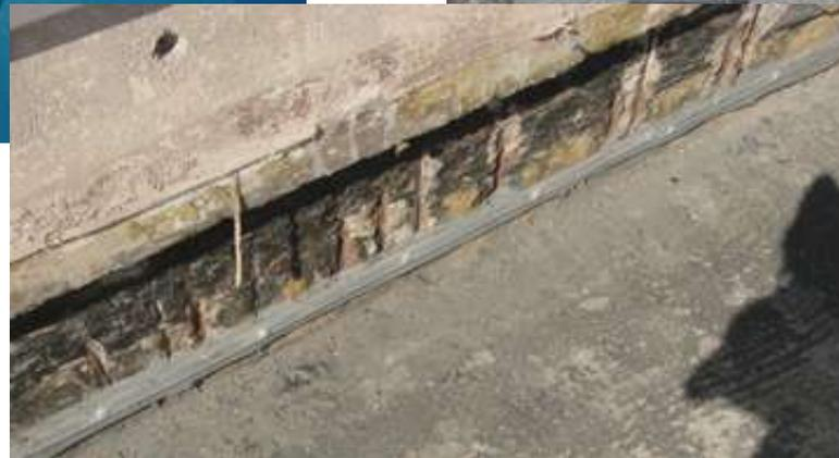
Corrosion Due to Carbonation and Low Concrete Cover over Rebar.
