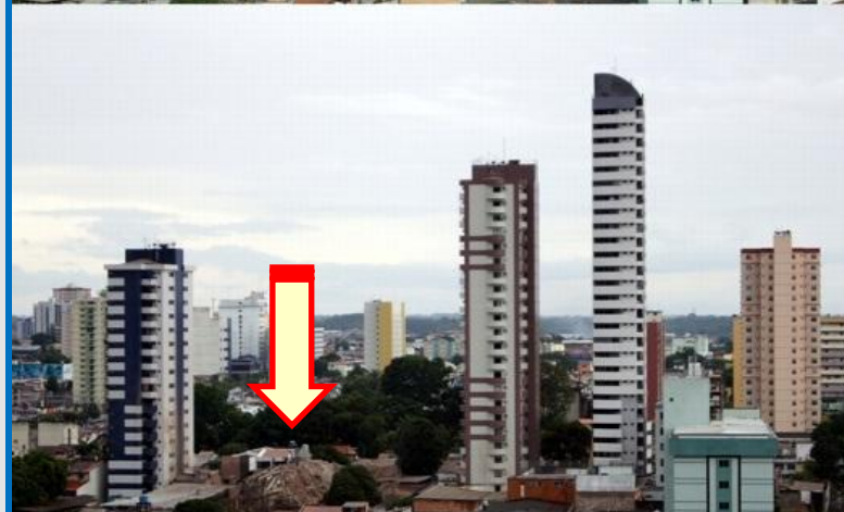
COLAPSO ED. REAL CLASS-BELÉM/PA
