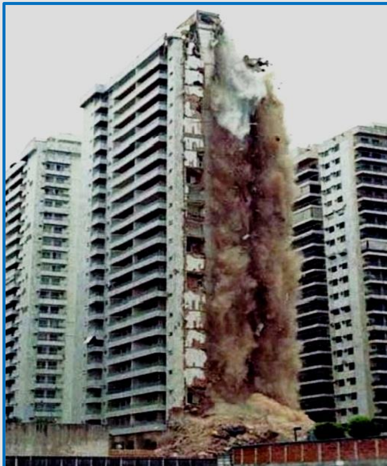
COLAPSO DO ED. PALACE II
