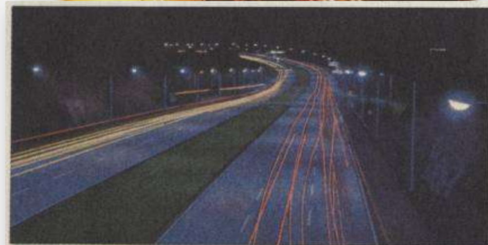
Concrete cuts highway lighting costs. Studies show proper lighting levels can be reached on concrete with 50% fewer fixtures than needed for dark-colored pavement.
