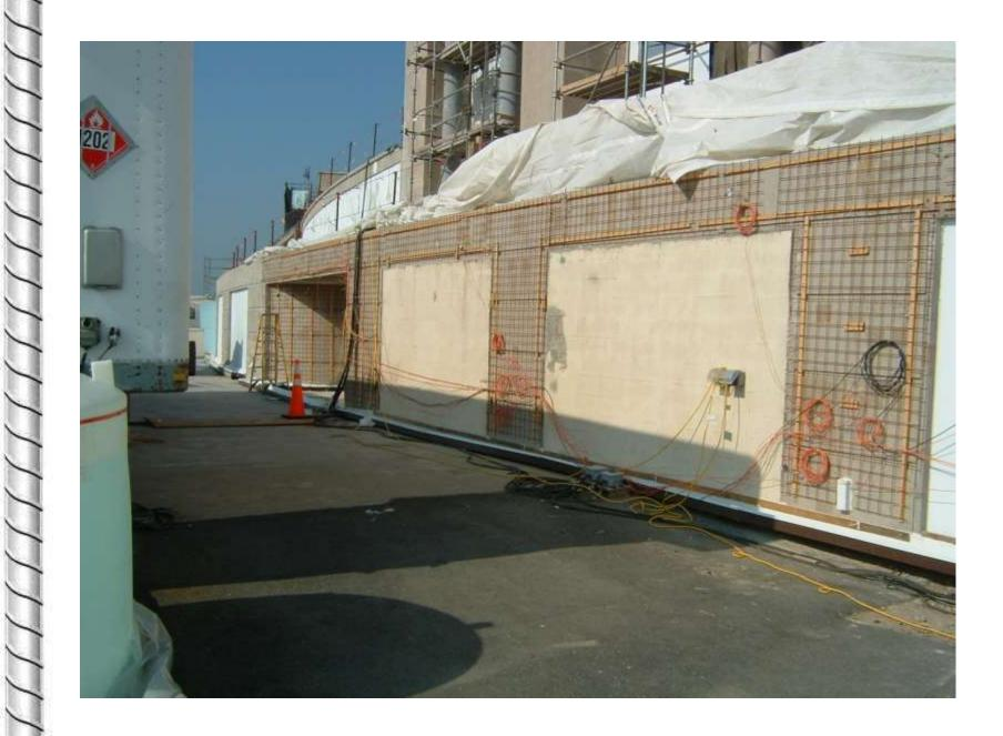
Norcure<sup>®</sup> Chloride Extraction and Re-alkalization of Concrete Facade.
