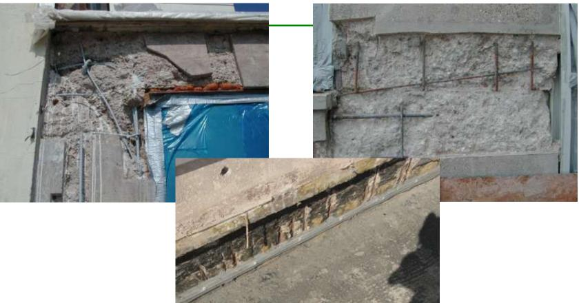
Corrosion Due to Carbonation and Low Concrete Cover over Rebar.
