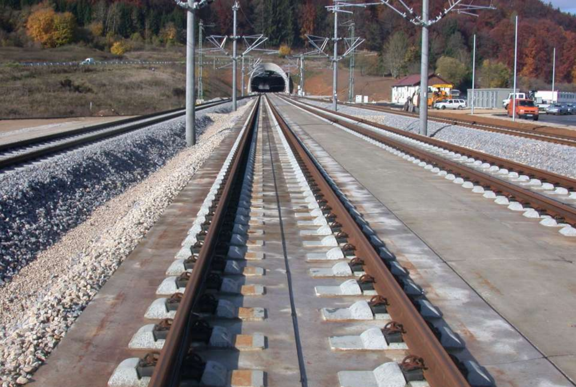
Continuously Reinforced Concrete Pavement for ballastless tracks (Nuremberg-Ingolstadt)
