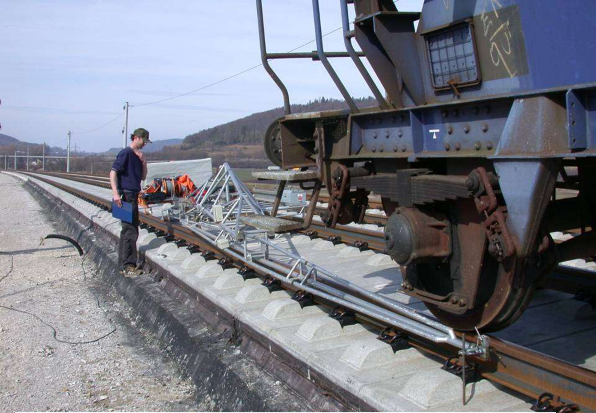
Track movable Benkelman beam to check track quality
