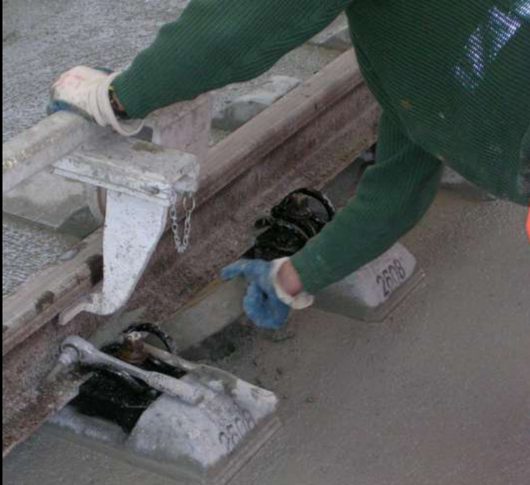
Temporary rail support removed
