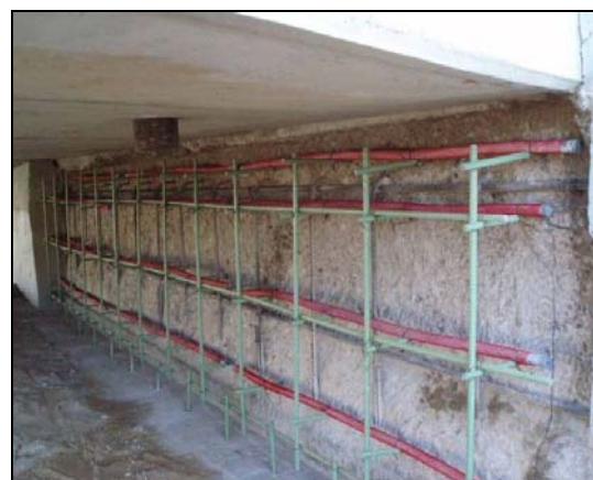
Figure 6: Distributed Galvanic Anodes (Red) Installed Prior to Concrete Placement
