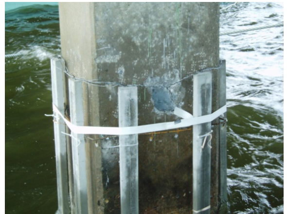
Figure 11: Distributed Anodes Placed Around NYSDOT Reinforced Concrete Pile Prior to Encasement
