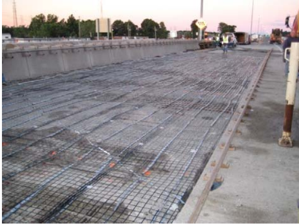
Figure 9: Distributed Anodes Installed on Ohio ODT Bridge Deck
