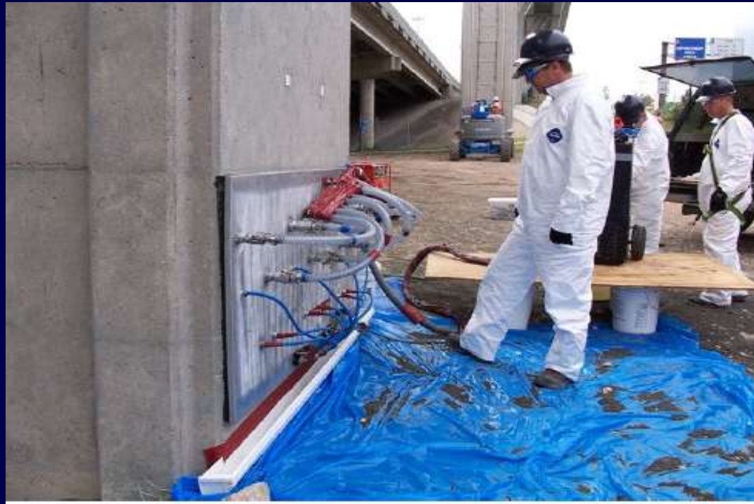
Vacuum impregnation \text{LiNO}_3
