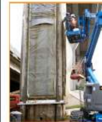
Electrochemical treatment on ASR-affected columns in Houston, TX
