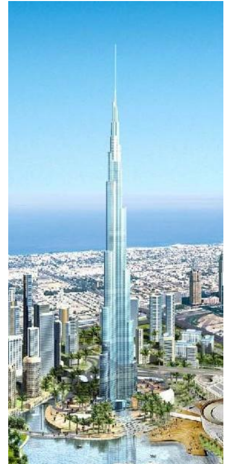
Burj Dubai “Dubai Tower” > 800 m (1/2 mile) [courtesy of wikipedia.org]
