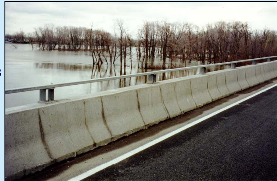
Vachon bridge, Laval, Canada, 1996 (a few days after rehabilitation)
