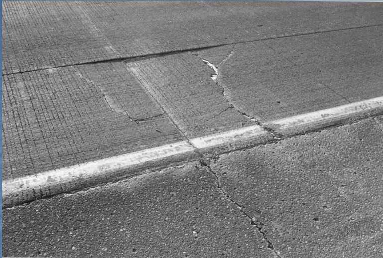
Transverse Cracking
