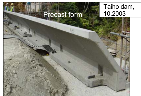
Photo 28- Set up of precast form
