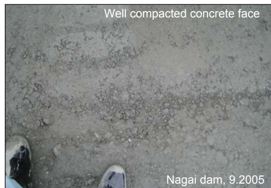
Photo 22- RCD concrete after compaction
