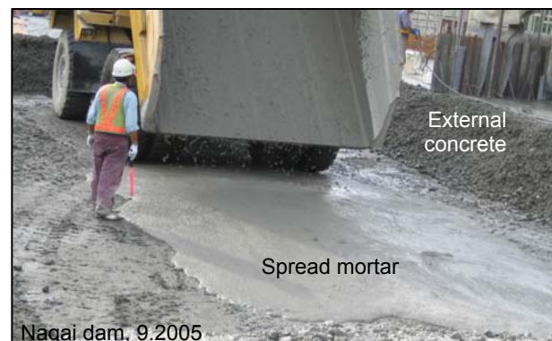
Photo 20- Lift joint treatment: mortar spreading
