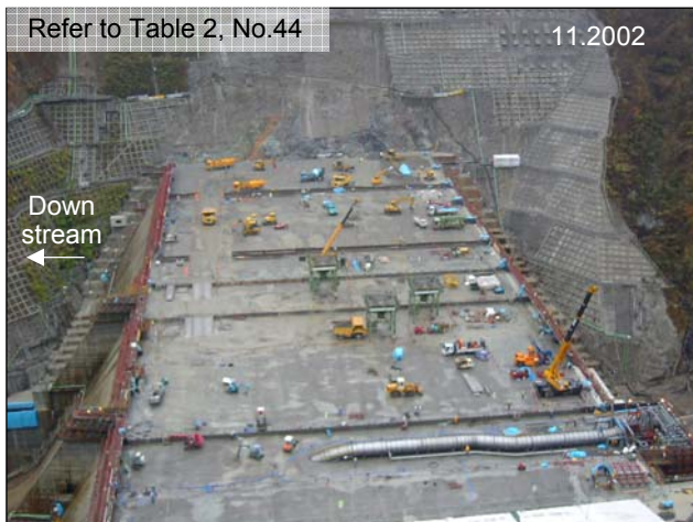
Photo 1 - RCD construction in Takizawa dam
