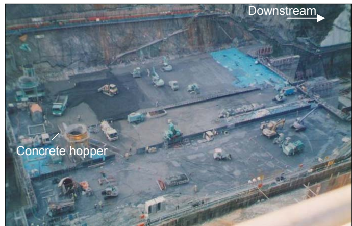
Photo 16 - Tower crane, Ueno dam, 11.1998
