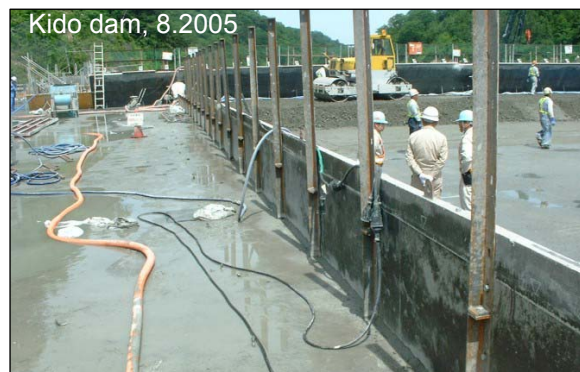
Photo 24- Block forms along the placing end
