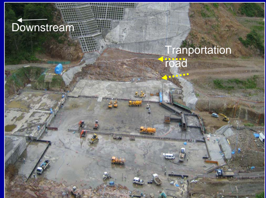
Dump truck, Toppu dam, 7.2005
