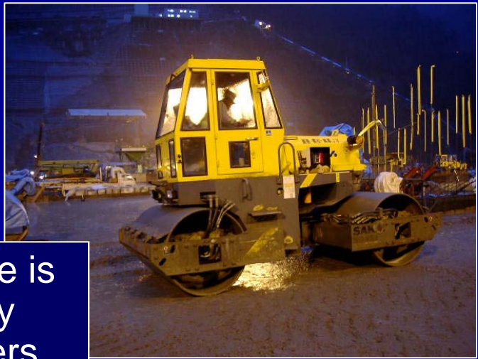
Vibratory roller, 11.2002, Takizawa dam
