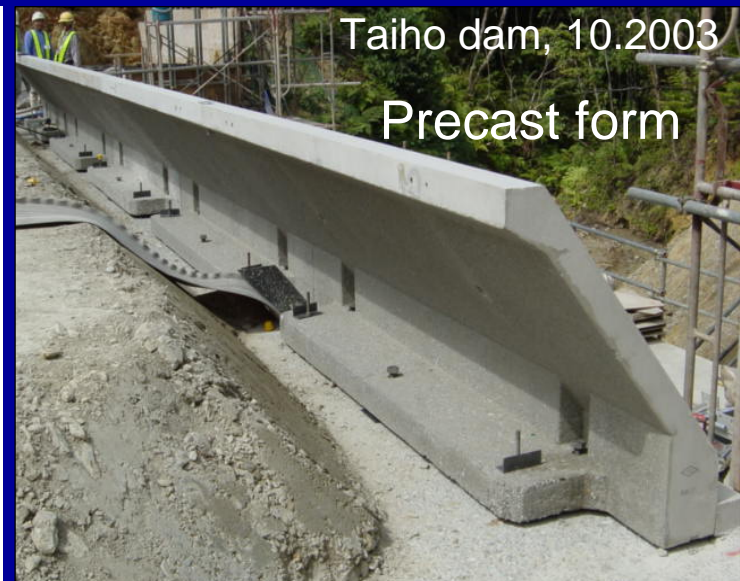
Set up of precast form
