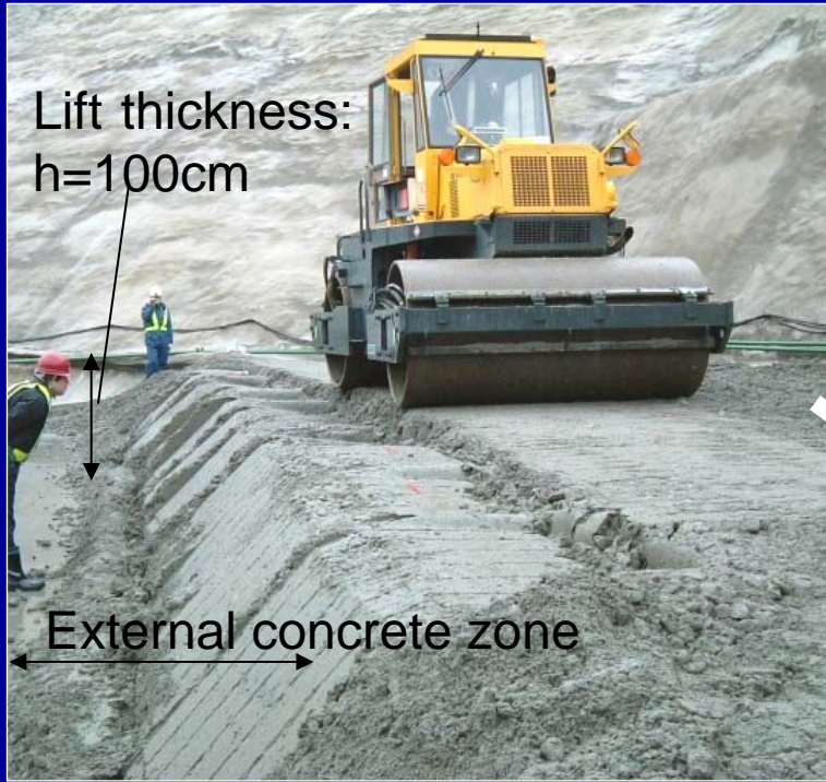
Internal RCD concrete
