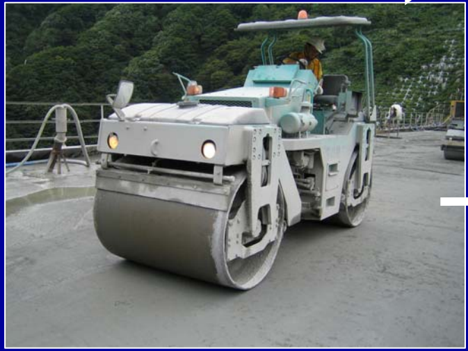
Finishing compaction by tire roller
