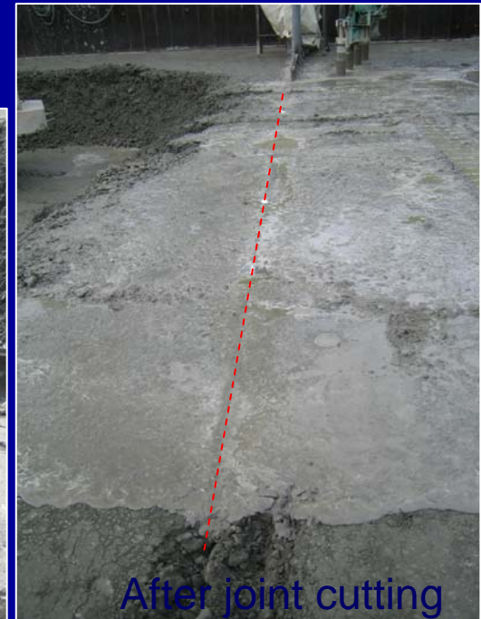
Contraction joints are cut by a vibratory blade machine
