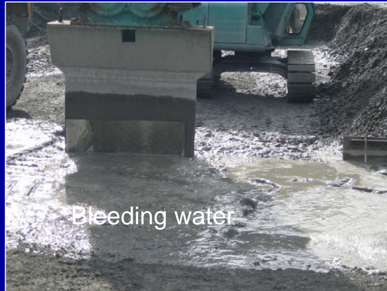
Contraction joints are cut by a vibratory blade machine
