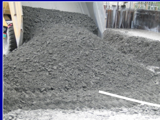
Unloading concrete
