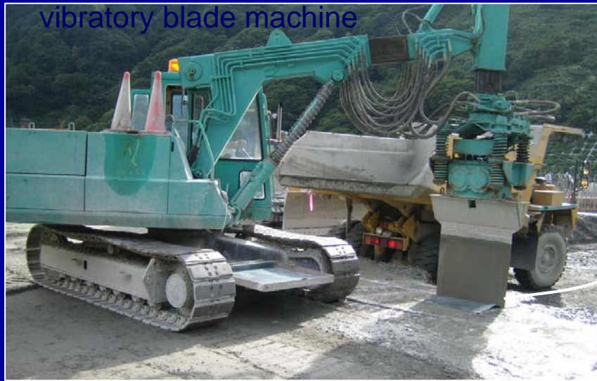
Contraction joints are cut by a vibratory blade machine
