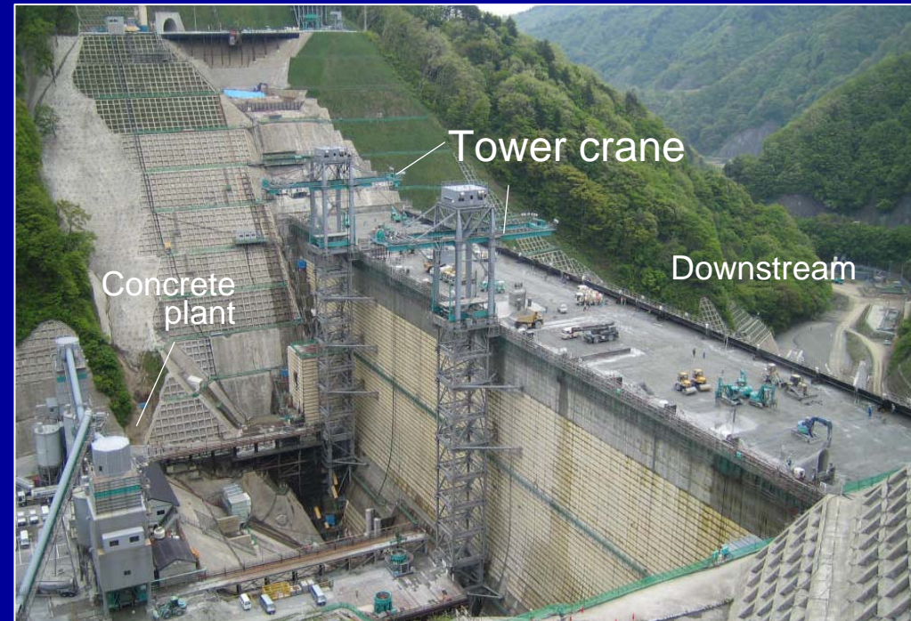
Tower crane, Nagai dam, 5.2005
