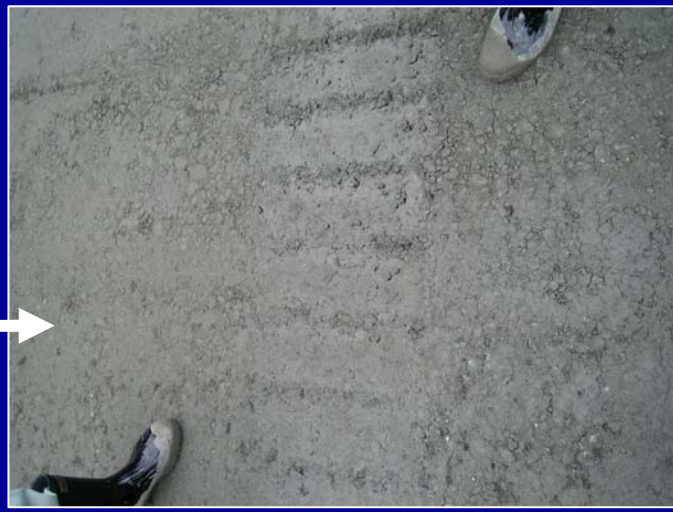
RCD concrete after compaction
