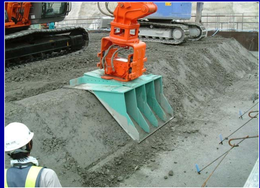
Well compacted internal end using a special machine
