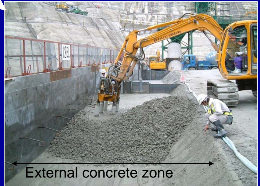
Well compacted internal end using a special machine
