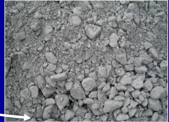
Segregation of large size Aggregate
