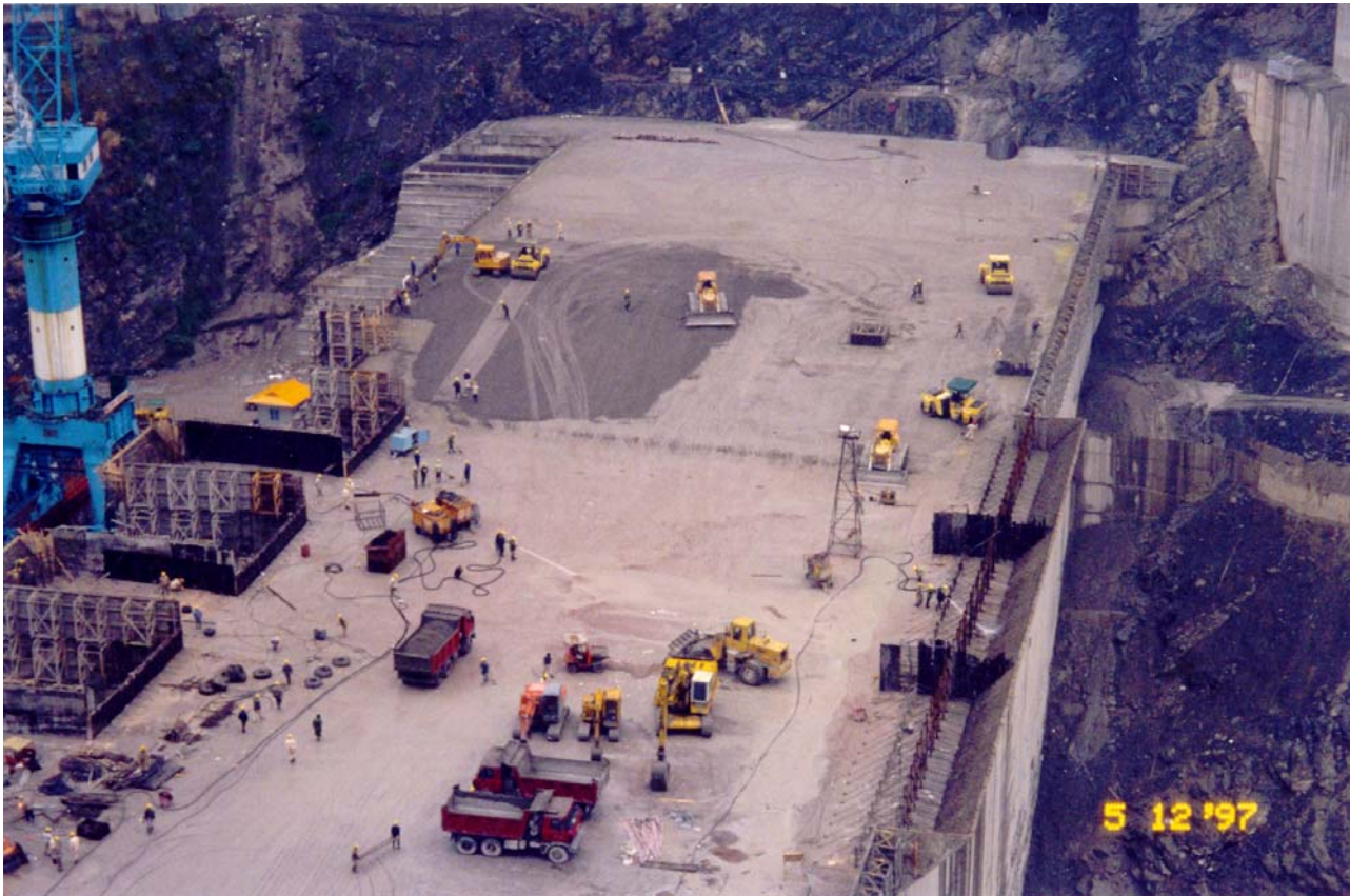
Photo 5 - Jiangya Dam showing the SLM using 3m high lifts
