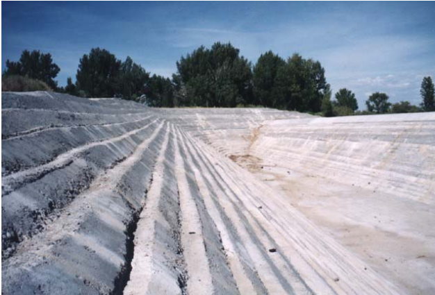
Figure 5 – RCC side channel spillway at Cold Springs Dam Spillway Modification (Bureau of Reclamation, 1996).
