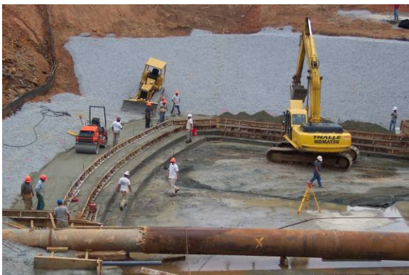
Figure 10 - Construction filter/drainage layer and first few lifts of RCC with formed edges (Golder 2003).
