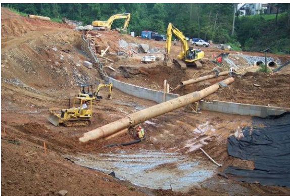
Figure 8 - Foundation preparation and construction of conventional concrete downstream cutoff wall at Y-14 (Golder 2003)
