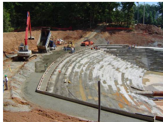
Figure 9 - Equipment used to haul, place, spread and compact the RCC (Golder 2003).
