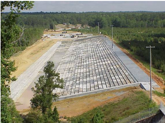
Figure 12 - RCC spillway and collection channel at Tholocco Lake Dam (USACE, 2000)
