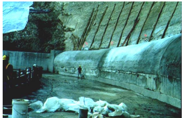
Figure 2 – Shotcrete gallery and buttress contact drains for Santa Cruz Dam (Bureau of Reclamation, 1990).
