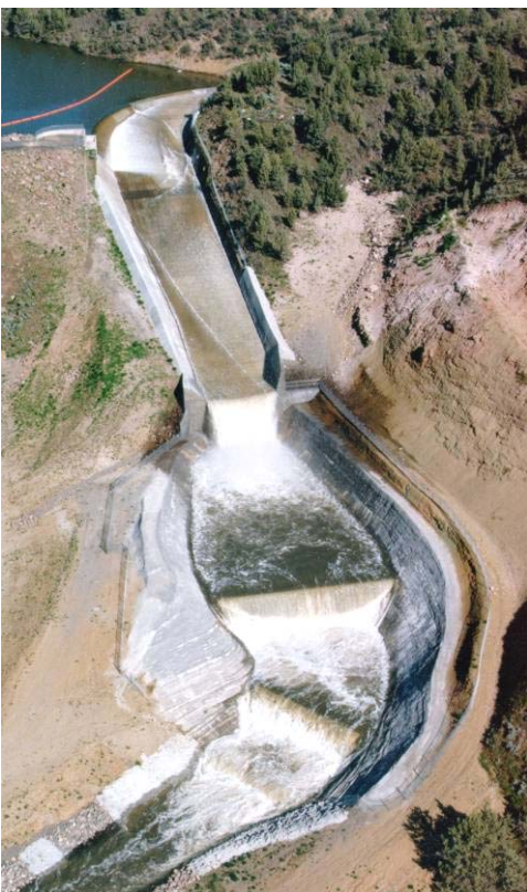
Figure 7 – Ochoco Dam Spillway Modification stilling basin plunge pool spilling during flood of record (Bureau of Reclamation, 1997).
