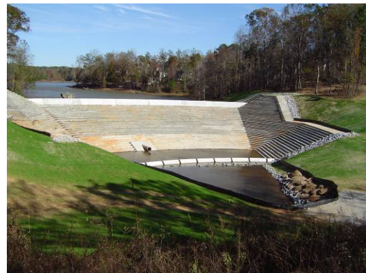
Figure 11 - Completed RCC Spillway with reinforced conventional concrete Ogee Crest (Golder 2003).
