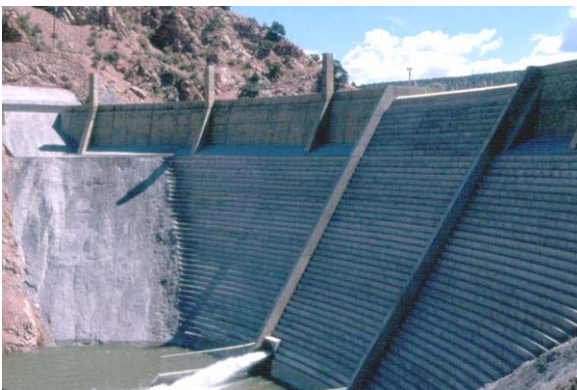
Figure 1 - RCC buttress with stepped facing for Santa Cruz Dam (Bureau of Reclamation, 1990).
