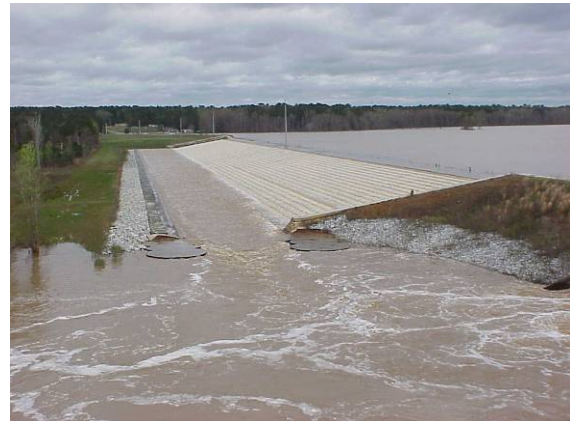
Figure 13 - RCC spillway during an overtopping event (USACE, 2005).
