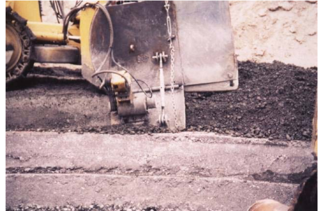
Figure 6 - Vibrating plate compactor for RCC edge at Cold Springs Dam Spillway Modification. (Bureau of Reclamation, 1996).
