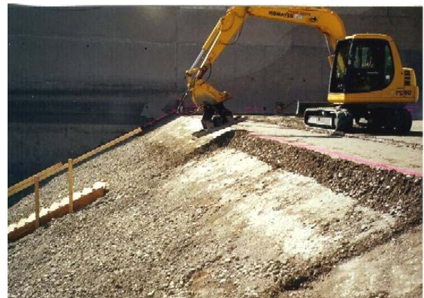
Figure 4 - Vibrating plate compaction of "toe block" at Pueblo Dam Modification (Bureau of Reclamation, 1998).
