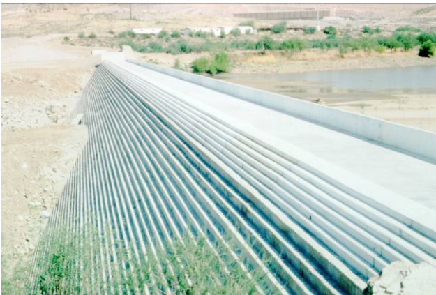
Figure 3 – All RCC stepped spillway at Camp Dyer Diversion Dam spillway after completion (Bureau of Reclamation, 1992).
