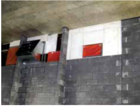
Figure 5 – Completed wall showing openings for ducting
