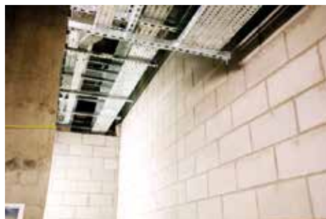
Figure 6 – Complex services at wall head
